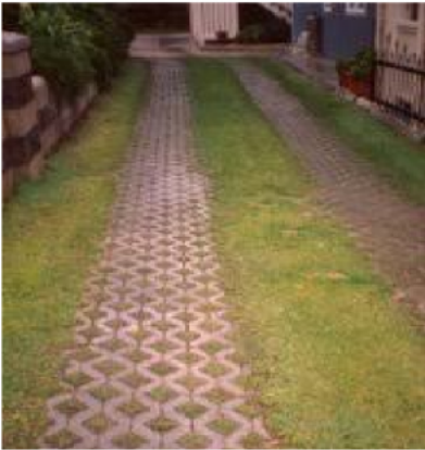
Some of Salix's work to reduce impervious surfaces on driveways
